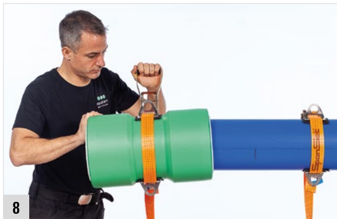
8 Final insertion of the pipe into the fitting must be done with an alignment tool.
