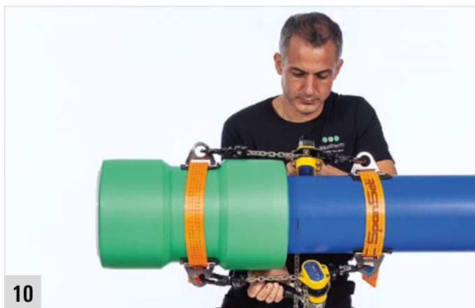
10 Pull the push-fit fitting onto the pipe end up to the marked insertion depth.
